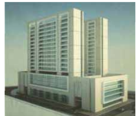
BOMBAY HOSPITAL- JAIPUR (Under Construction)
